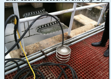
Fig. C. Sieve set up at the Plattsburgh WWTP. Gives a view of the open channel at the end of the waste treatment process.
